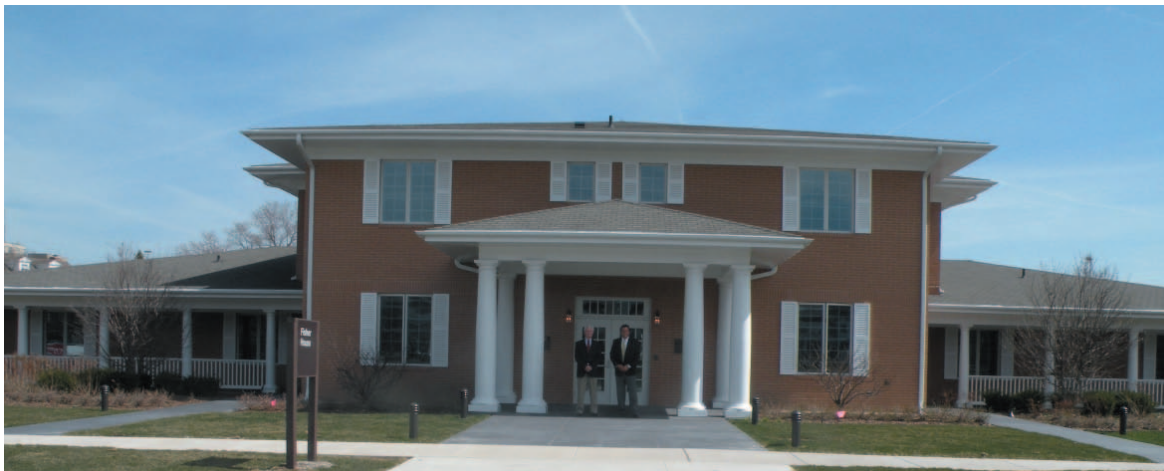
The new Fisher House at Hines VA Hospital. Sam Lazich and Bill Anderson, DMS Pharmaceutical Group, took a pre-grand opening tour of the house and provided the photos included here.
